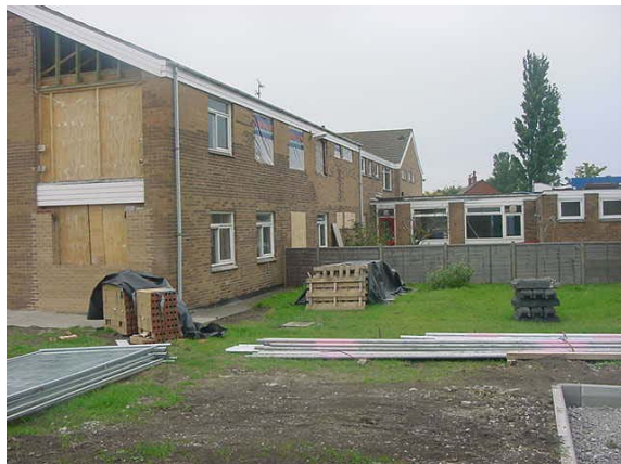
The premises can be seen under refurbishment
