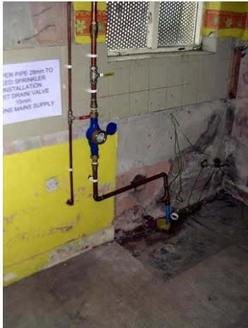
Fig 4 Supply inlet and flow meter
