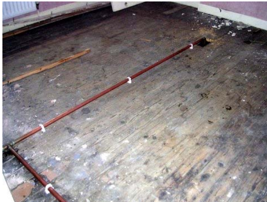
Fig 5 The pipe installation above the lounge
